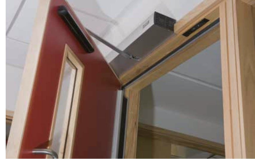
Motion sensor controlled power operated door
